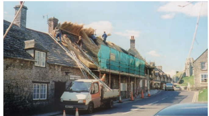
Thatching a roof in Dorset, UK – an ancient skill possessed by a relatively small number of tradespeople today.
