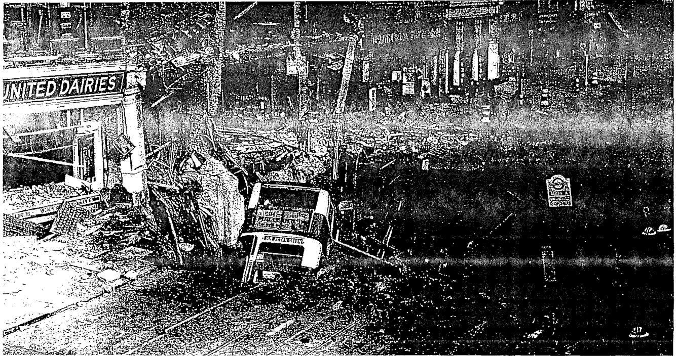
Balham High Street, South-West London, 17 October 1940. As well as wrecking buildings in the street, this bomb explosion destroyed the sub-surface gas, electricity and water mains. This flooded the underground railway station beneath the street, killing sixty-three people sheltering there
