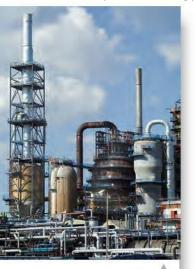
Catalytic cracking uses high temperature and a catalyst to break down (crack) heavy oil fractions into lighter, more useful oils. The oil is heated to 500 °C and passed over a catalyst such as zeolite crystals. The vessel where the cracking takes places is the barrelshaped grey one on the right.
