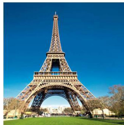
The Eiffel Tower is constructed from a lattice that contains thousands of triangles.
