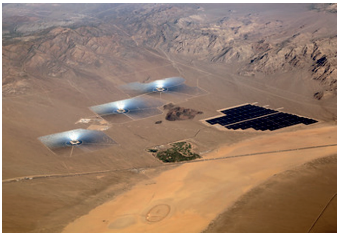
Figure 8(c): The Ivanpah Solar Thermal Plant and Desert Sunlight Solar Farm cover an area of 29 km 2 in southern California
