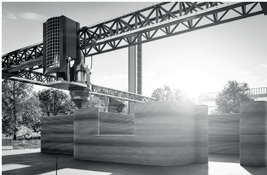
Figure 1: Artist's impression of a 3D-printed house in progress
